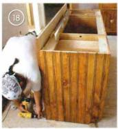
so checked the distance to the other cabinets. The corner cabinet was left loose with the idea that I could slide it up and out of the way when the countertop was installed and then drop it down for a precise fit on the granite counter.
